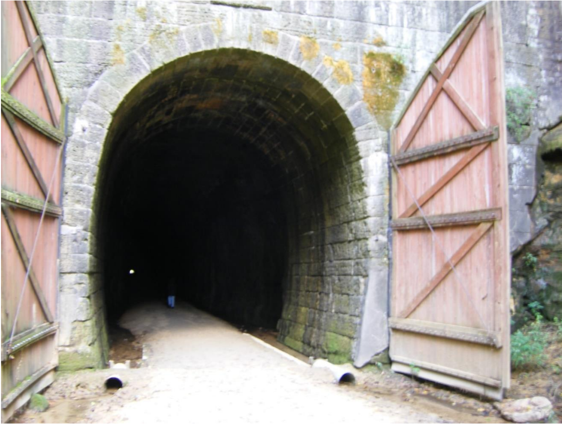
The tunnel entrance!
